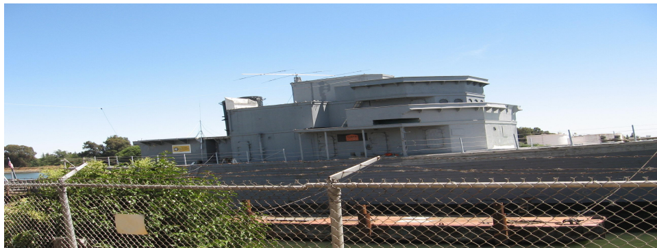
The USS Lucid undergoing restoration at the Port of Stockton. The 20 meter beam is on top of the superstructure.
