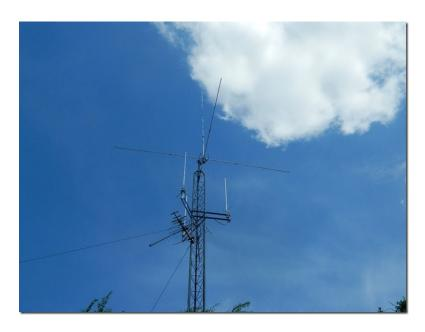
The ten meter ground plane is at 45' and the UHF/VHF verticals are at 34'. Other antennas include TV, FM broadcast and 900 MHz.
