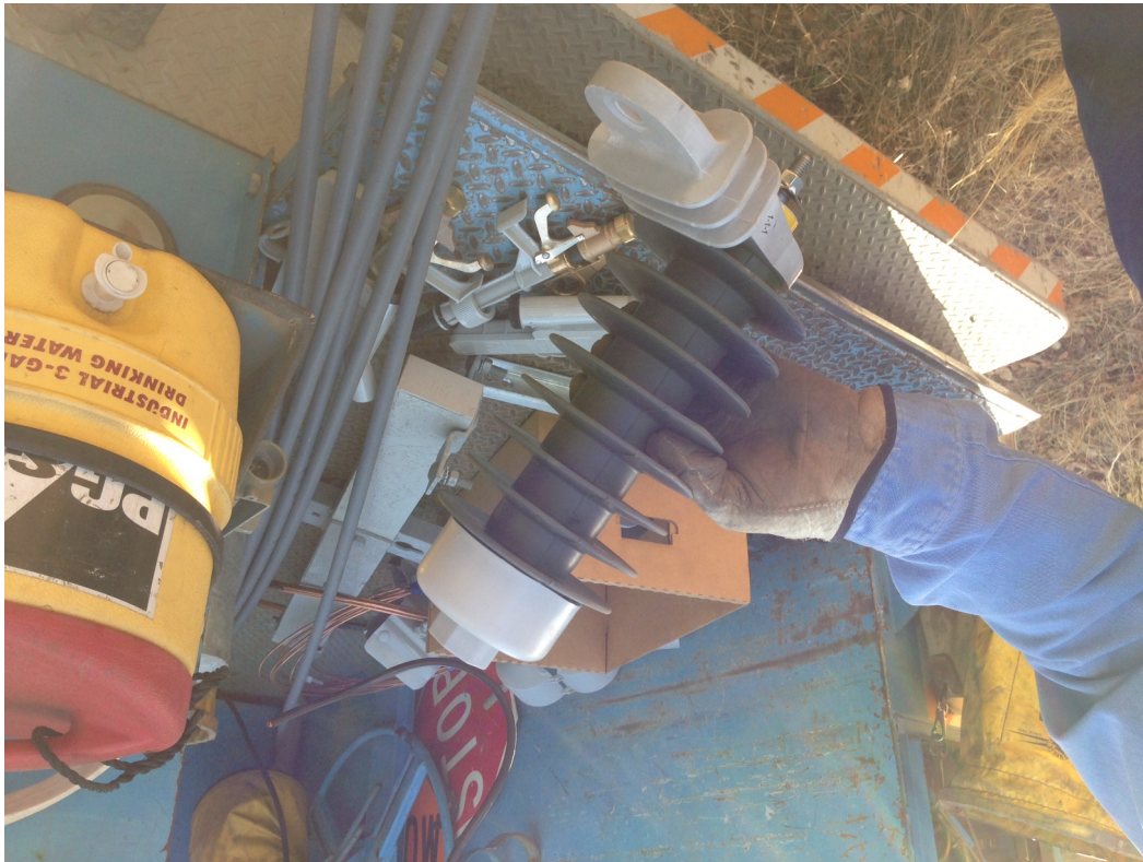
New Lightning Arrester
