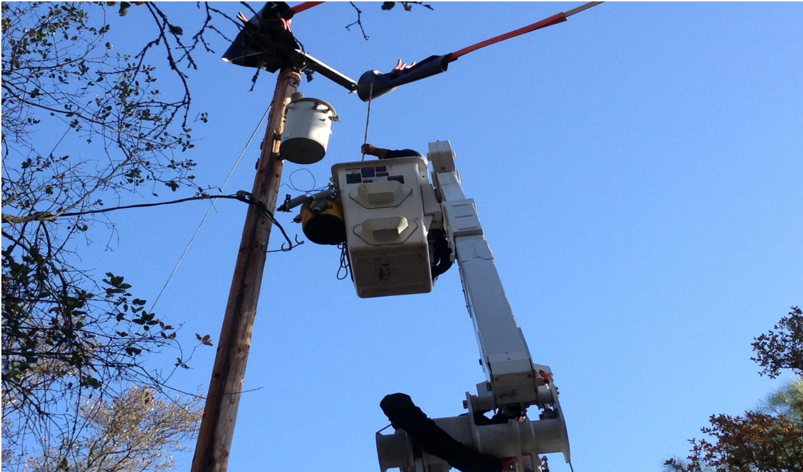
PG&E Boom Truck and Crew Removing Old Hardware
